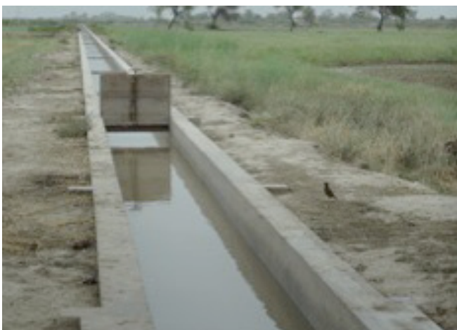
Al Dahra concrete made water course in village Syed Ali Nawaz Shah
